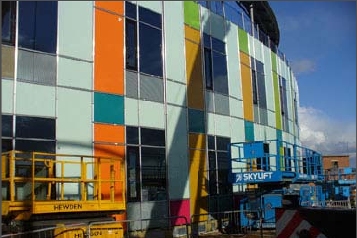
Women and Children's Unit with coloured glasses that create the external façades of the new buildings across the site.
