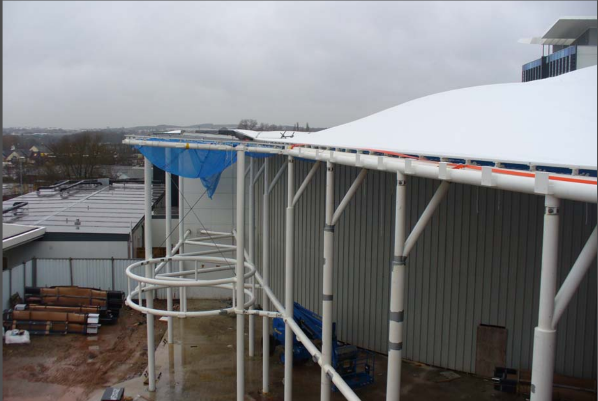
View of the main entrance.
