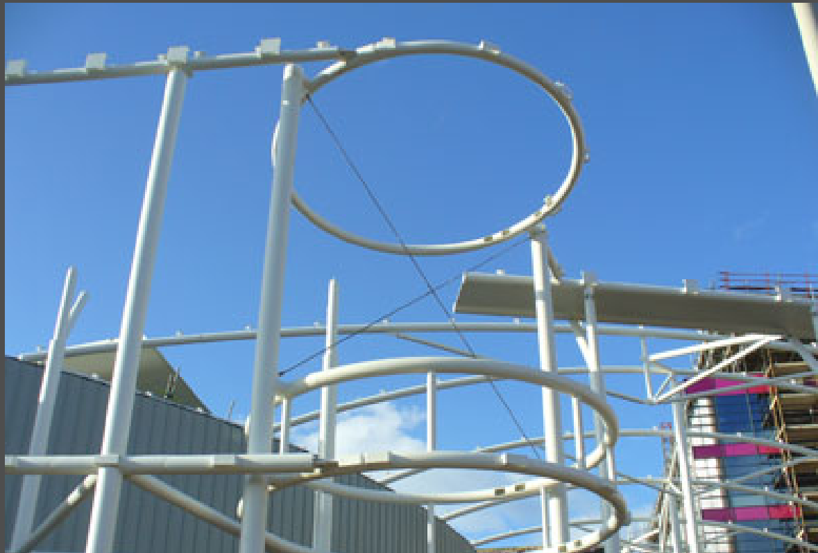
Steelwork in position for the main entrance door.
