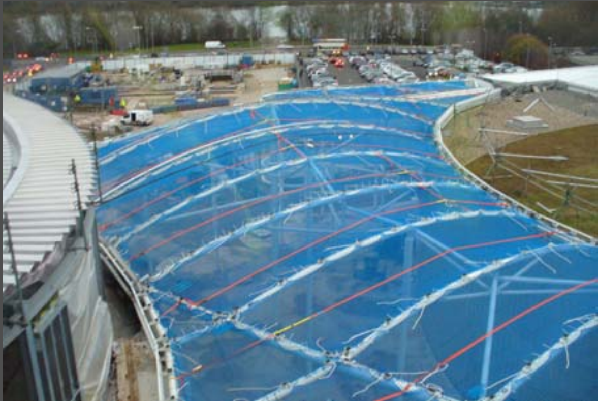
The roof structure and form of the new main entrance.
