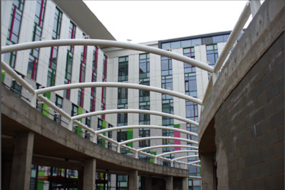
Skeleton roof over the retail area.
