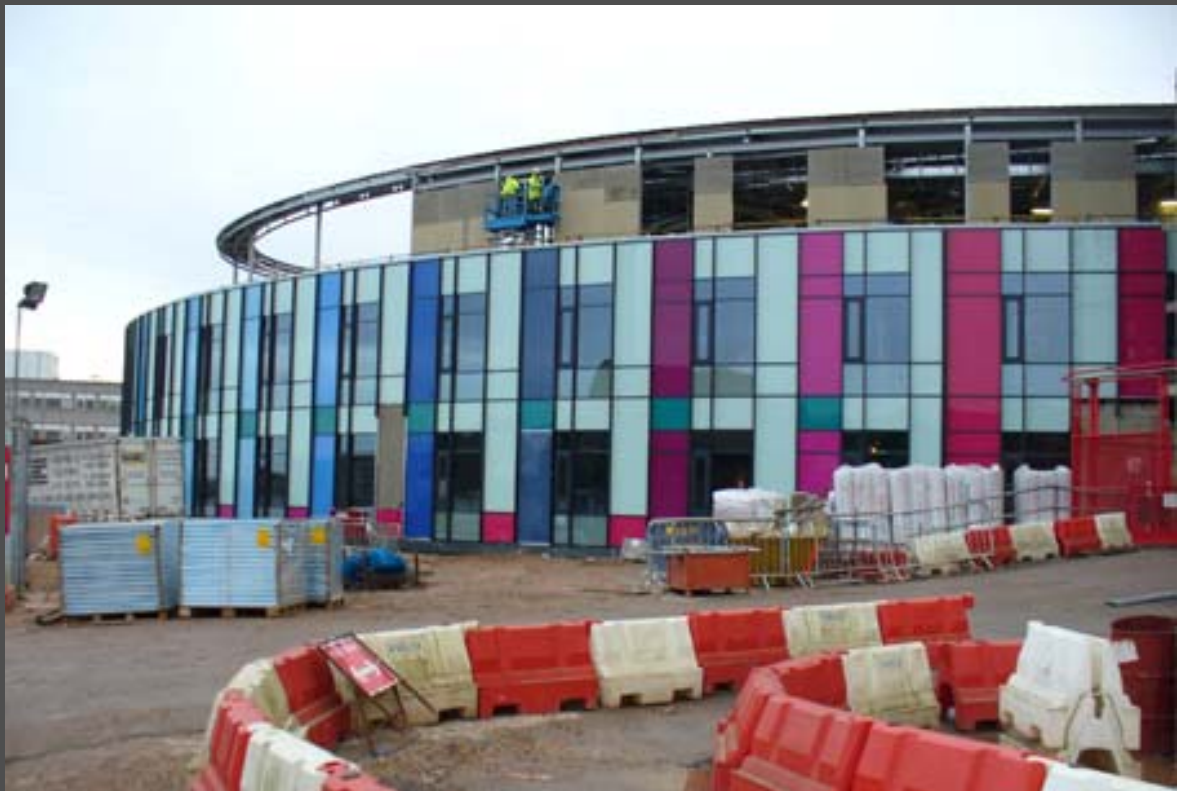
The side elevation of the Women and Children's unit.
