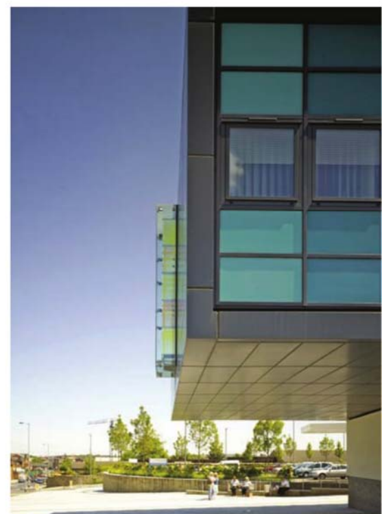
Dichroic glass blades on the first floor glazed bay at the end of the cantilever, refract light and change colour depending on the viewing angle and lighting conditions
